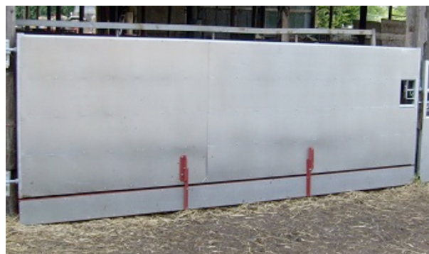
Fig.1: Adjustable flap on gate across cattle shed
