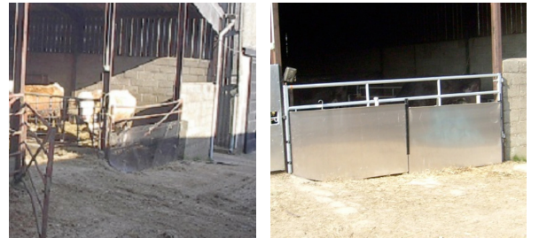
Fig.4: Cattle Shed (Before) Fig. 5: Cattle Shed (After)
