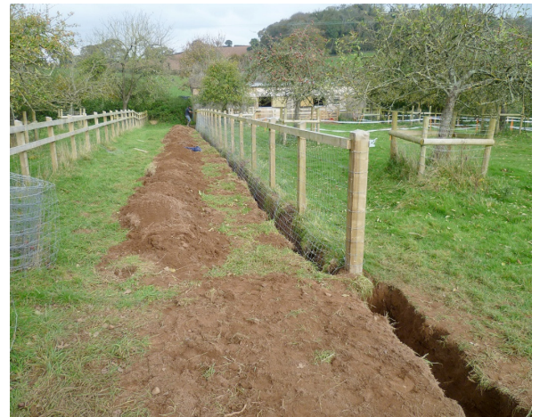
Fig. 2: Wire mesh fencing
